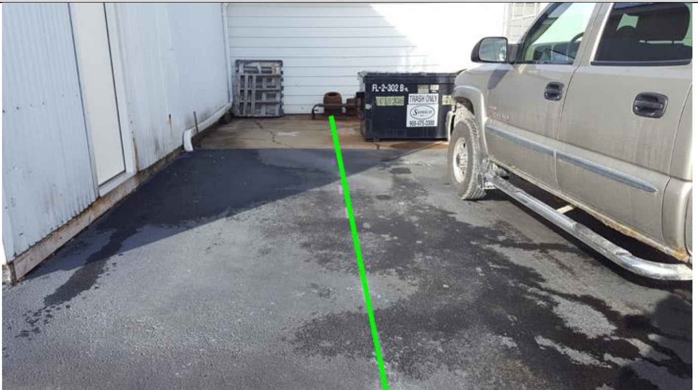
Northwest facing photo shows the storm sewer line which passes underneath the building and emerges on the back side.
