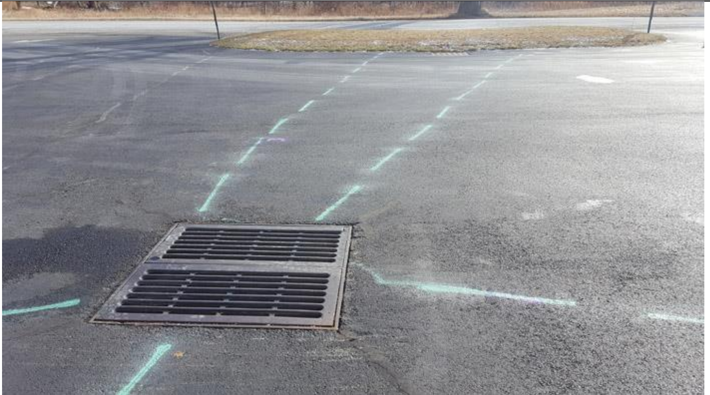
Southeast facing photo of the central sewer grate shown in Photo 14.
