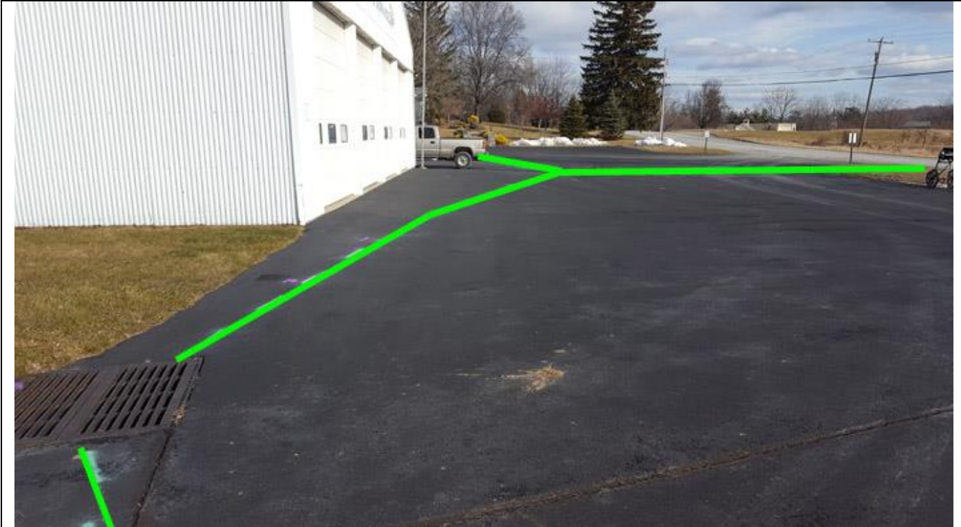
Northeast facing photo shows the storm sewer system beneath the asphalt. The sewers sit at depths of 3-4'.
