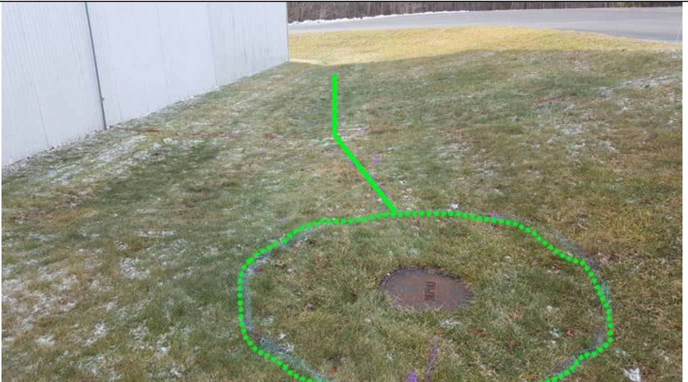
Southwest facing photo shows the circular concrete septic tank and the lateral PVC line that leads away from it. The lateral coincides with a topographic trough which is apparently filled with gravel.
