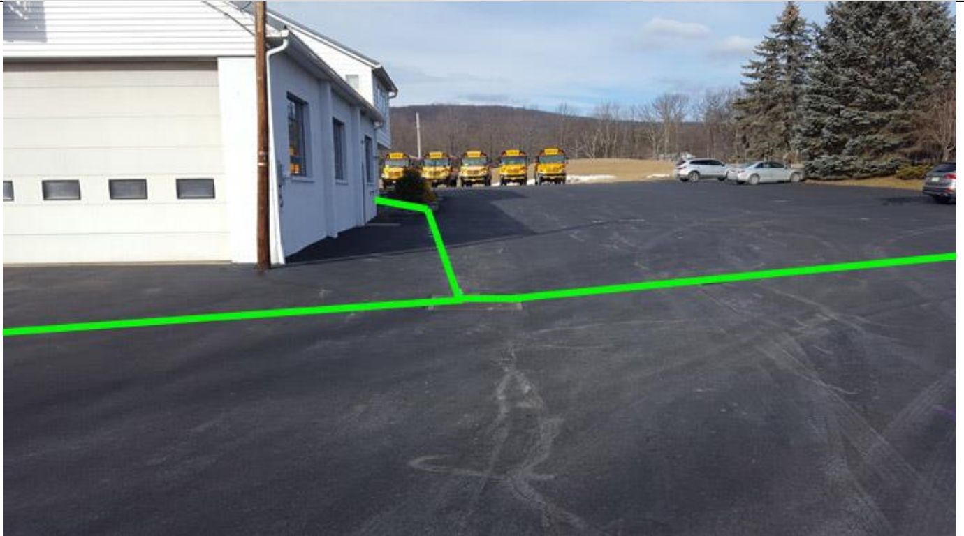
Northwest facing photo shows storm sewer lines.
