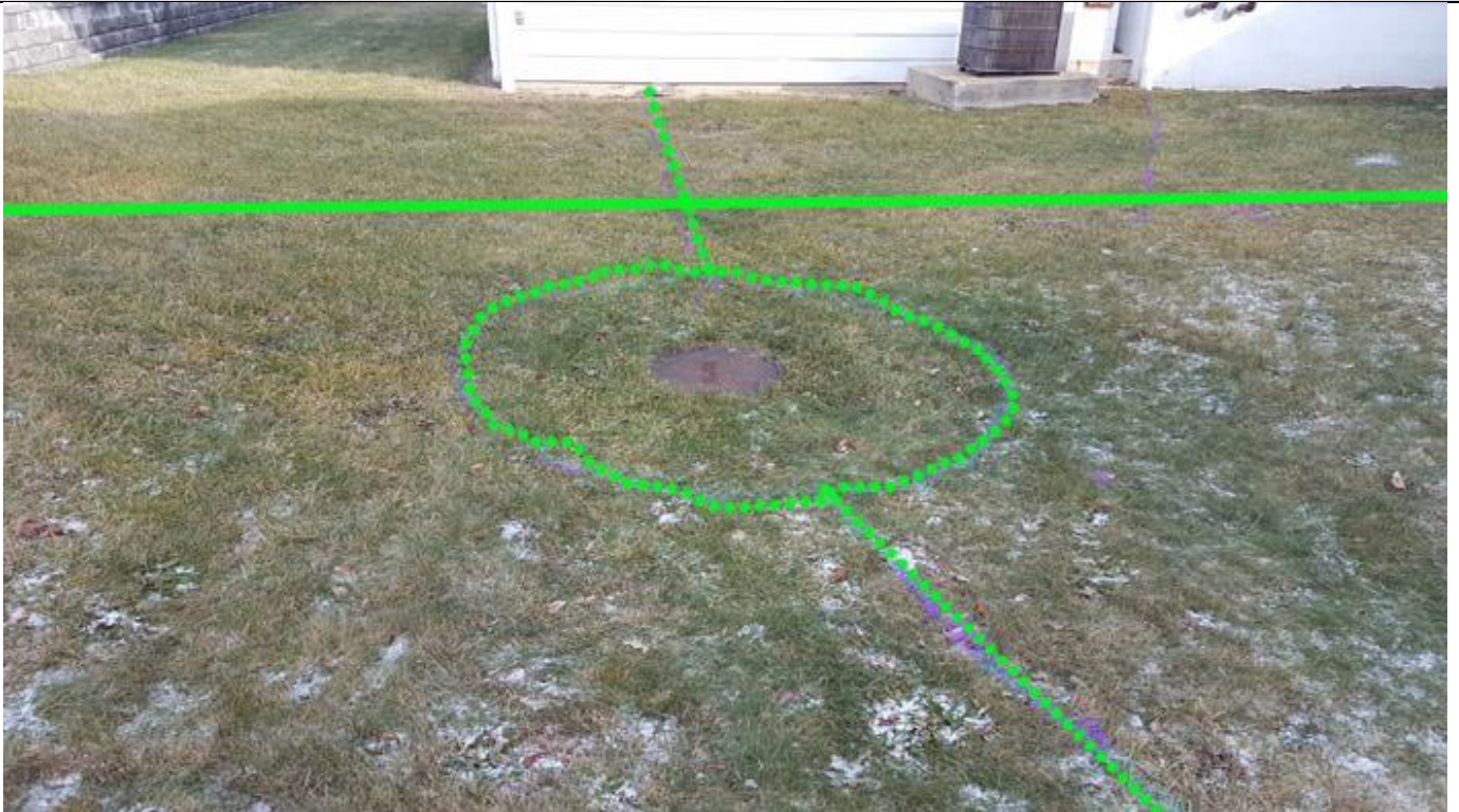
Northeast facing photo shows the circular concrete septic tank measuring around 6' in diameter. A sewer line conveys wastewater from the building to the tank. The lateral is in the foreground. The solid green line is a NW-SE trending storm sewer that goes beneath the building.
